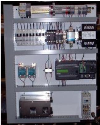
This is the third system that I built that uses this new P.L.C. by [Automation Direct.com](#) Its the [DL06 PLC](#). This panel controls a process that has 4 Temperature control zones and 4 analog sensors. Plus connection to the plant Ethernet.
