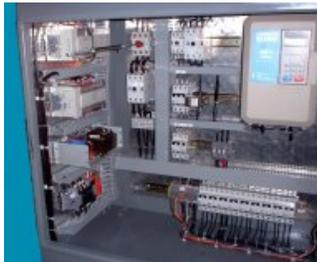
Here you can see the power distribution contactors and the 10HP
